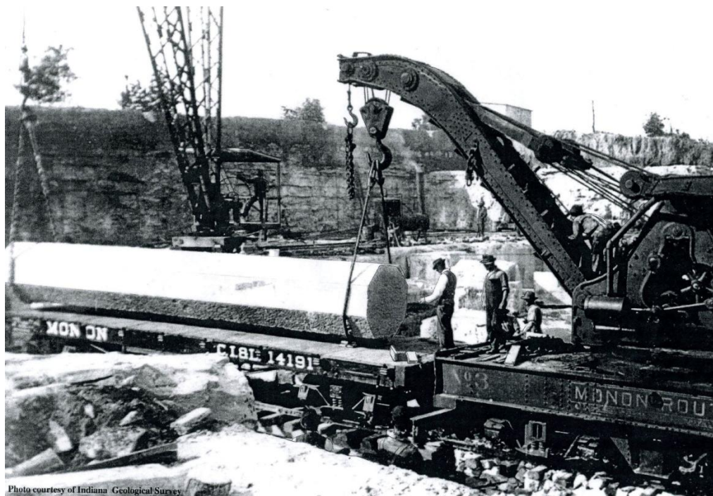
Fig. 14 The caption for this picture from David Hoadley's History states that the column is 37 feet long and 4 feet and 4 inches in diameter and weighs more than 50 tons.
