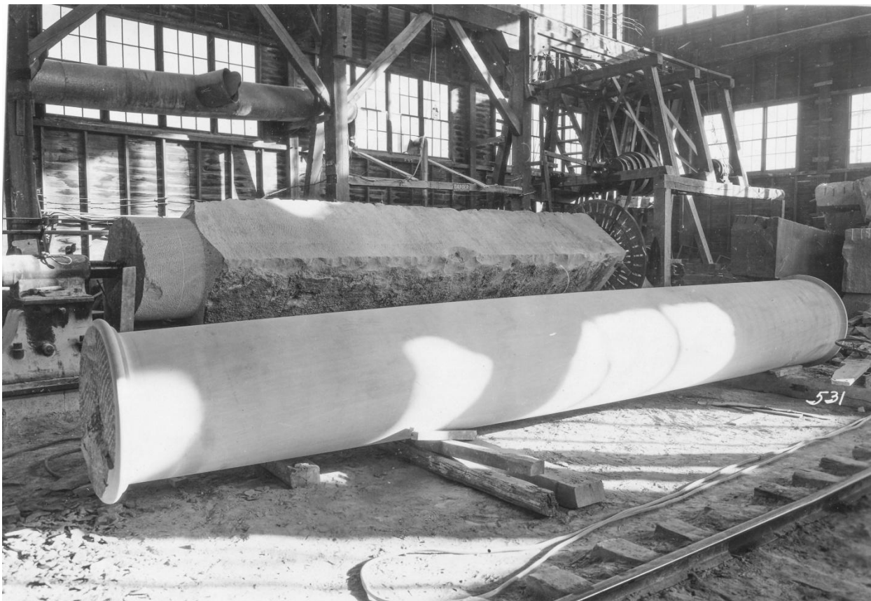
Fig. 11 This photo from John Tucker illustrates the before and after condition of a block of stone as it first comes from the quarry and the scabbling mill that removes most bulk stone. The lathe at the mill takes that and turns the column into its final form. This lathe was in the Consolidated Stone Co. Dark Hollow Mill.
