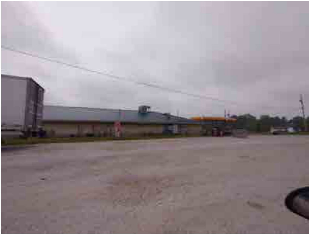
Figure 4: Looking southwest at the back of the convenience store.
