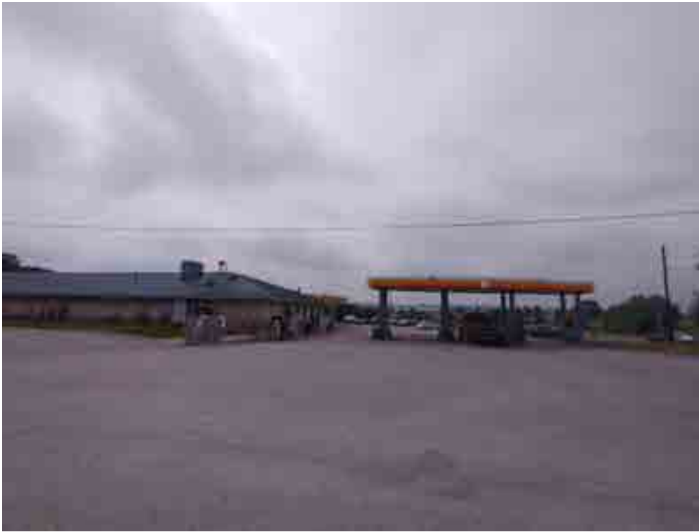
Figure 6. Looking south at one of two canopies.
