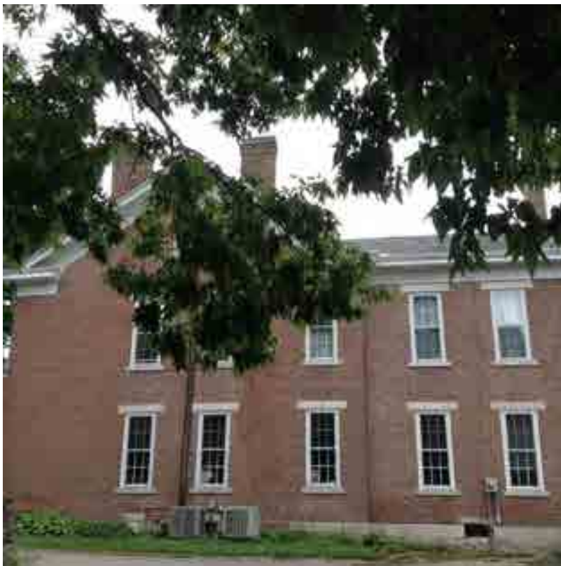
Photo 12: Existing single family residence
