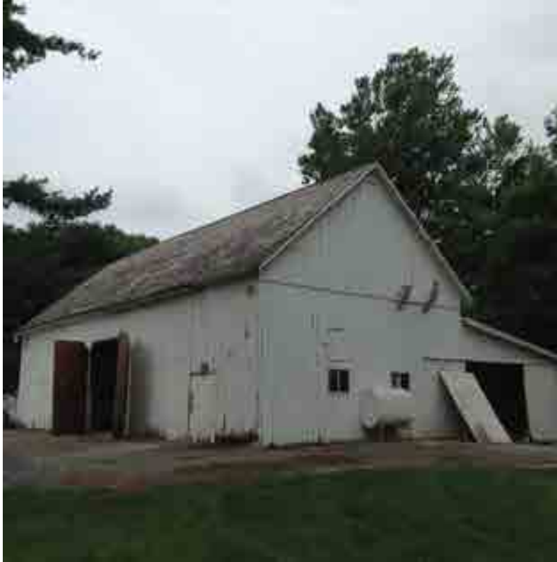
Photo 9: Barn to be renovated
