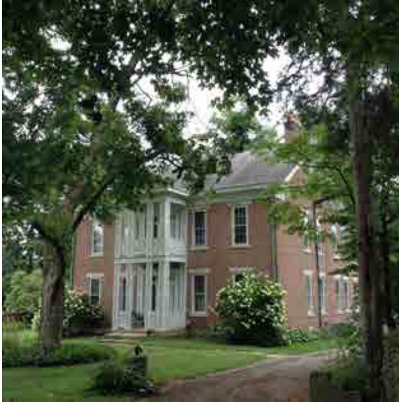
Photo 11: Existing single family residence
