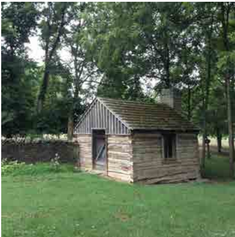
Photo 18: Original log cabin
