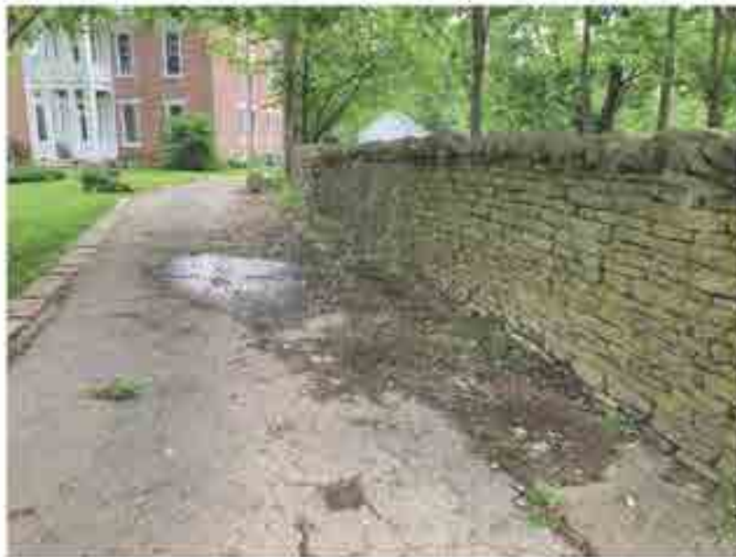
Stone wall along the driveway
