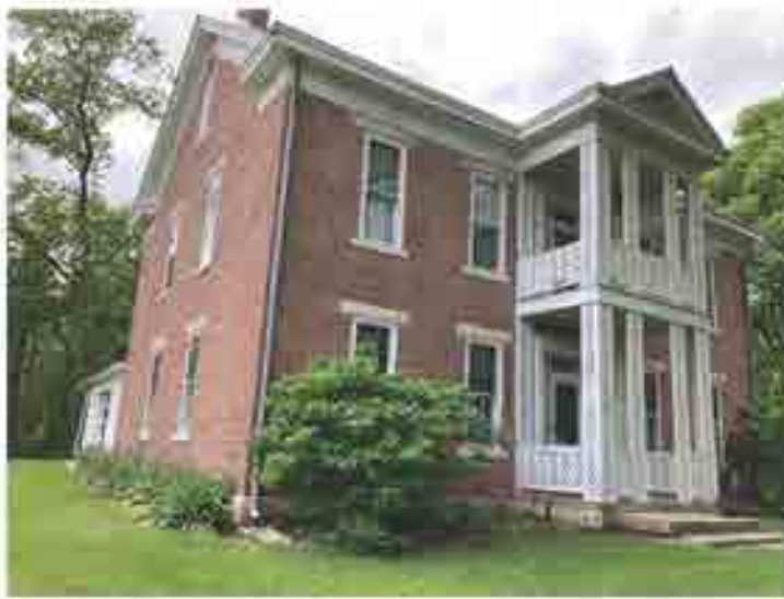
Front exterior of the home
