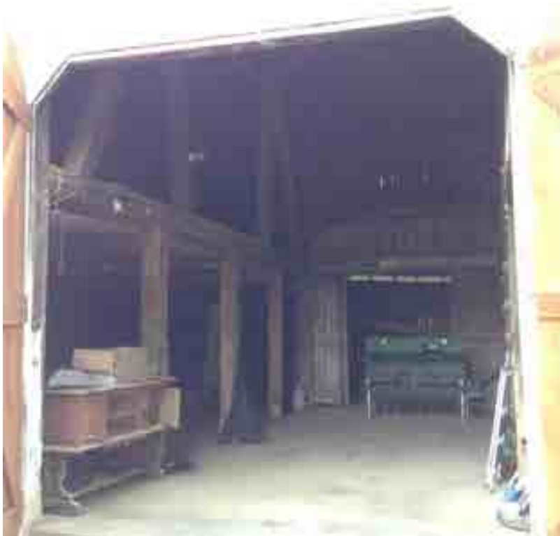
Photo 10: Inside barn to be renovated
