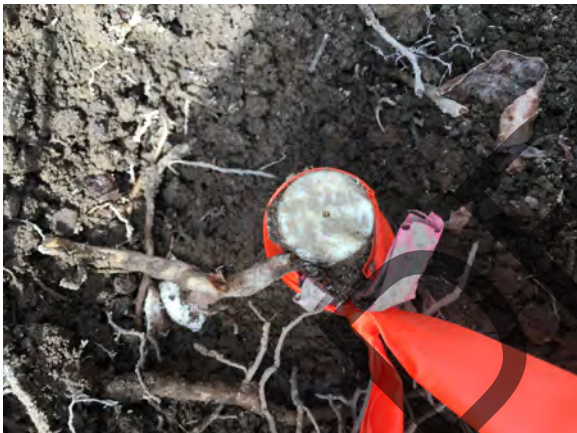
Photo Orientation & Description: Prall pipe at O25
