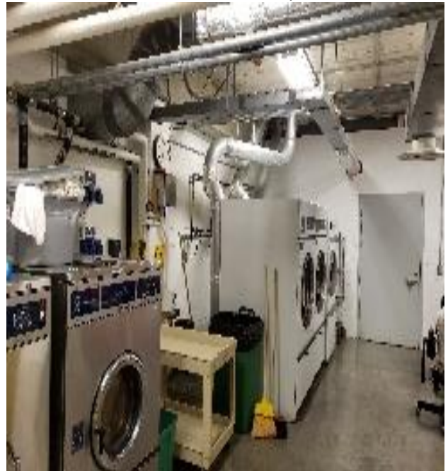
Exhibit V.5. Drafts and Dryer Vents
