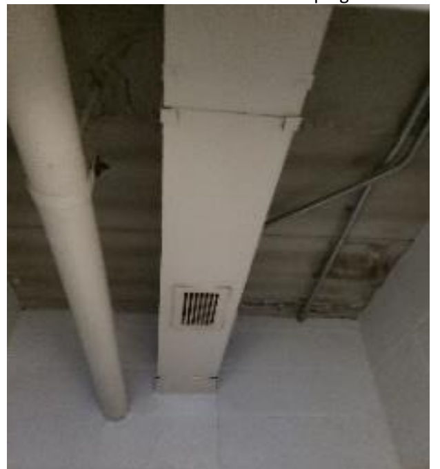
Exhibit V.7. Fasteners and Piping
