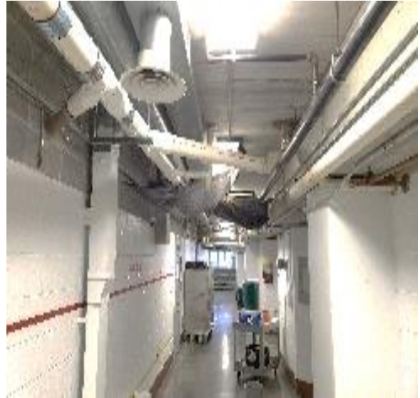
Exhibit V.25. Sprinkler Heads & Pipes
