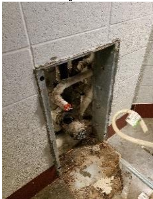
Exhibit V.22. Plumbing Fixtures & Isolation Valves
