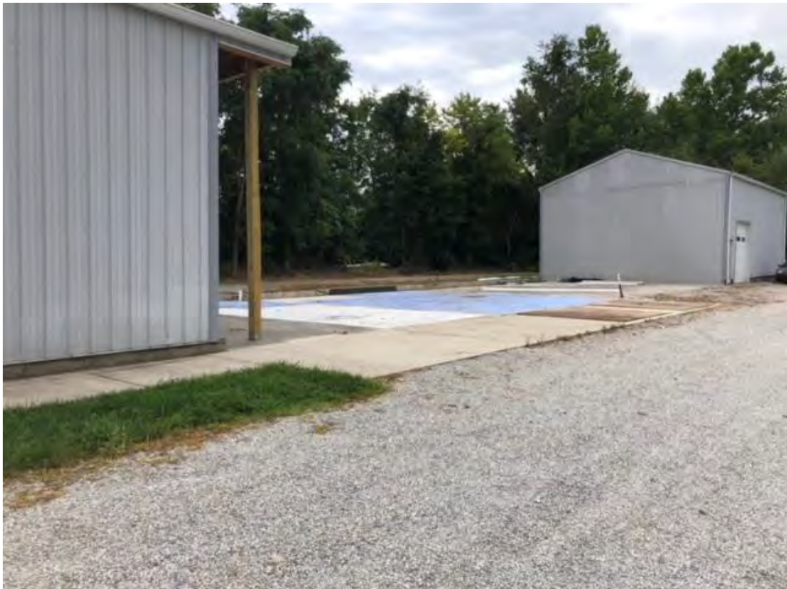
Photo 4. View of the buildings with the area in between no longer present August 2020. Photo by the Building Department.
