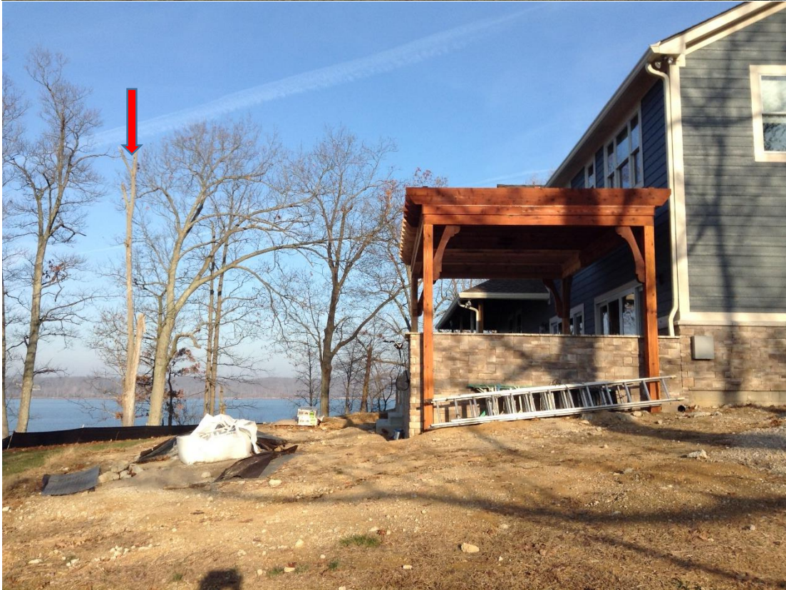
Figure 4. New 495 sf porch and 1,100 sf addition (2020). Silt fence was added after a majority of the project was completed.
