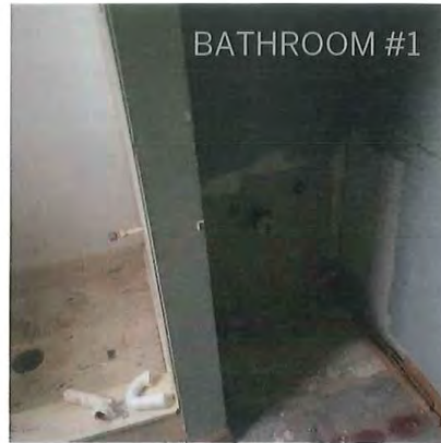
remove sink/shower fixtures and cap off
