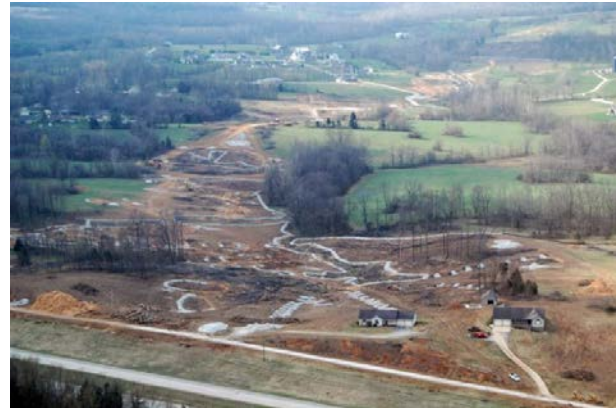
I-69 under construction
