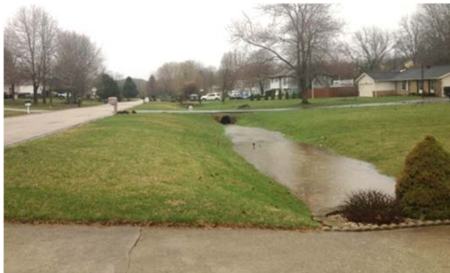
Cherry Lane surface drainage
