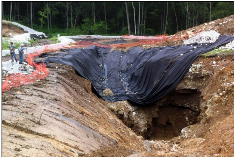
Sinkhole excavated and later filled with crushed limestone
