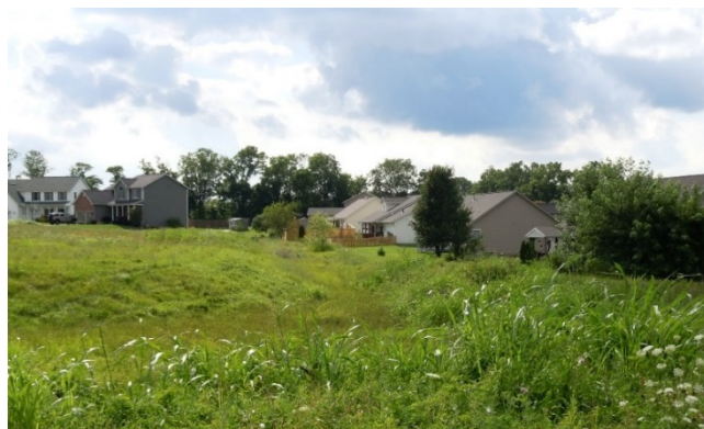
Stonechase subdivision detention pond
