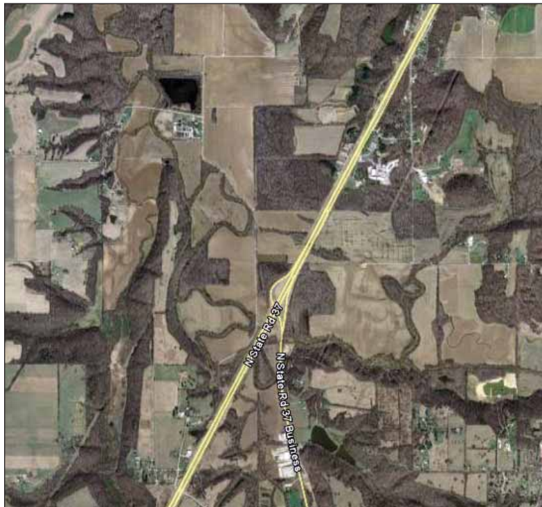
Figure 10: SR 37 in Monroe County. Source: GoogleEarth
