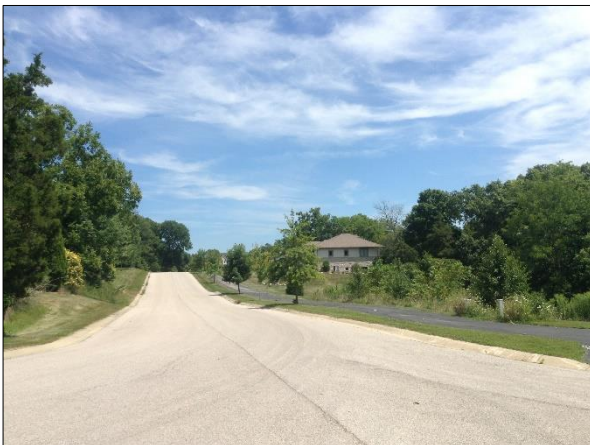
A sidepath is a hard surface path physically separated from the road by a grass or tree plot.
