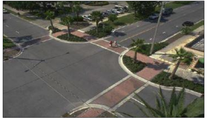
A crossing design that has curb bump-outs and special paving to improve pedestrian safety and wayfinding, while calming traffic.
