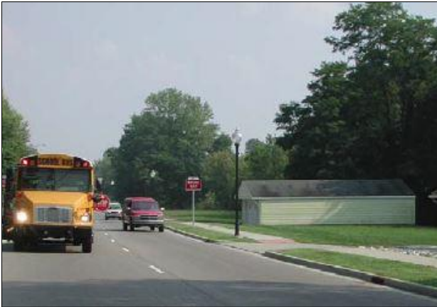
An urban collector sidewalk is a hard surface path along an arterial street with curb and gutter.
