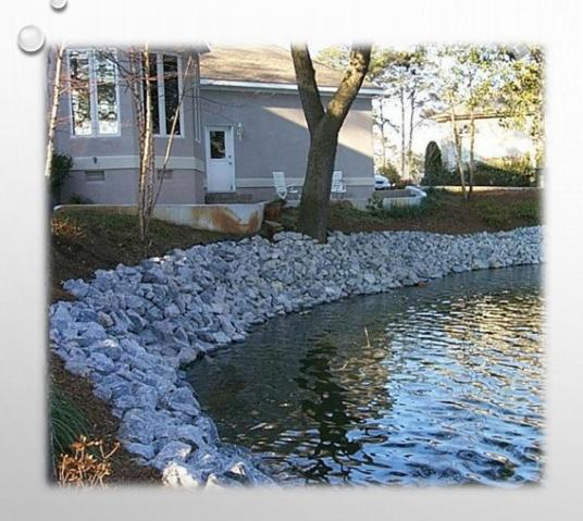
Surface stabilization placed on a vegetated slope to <u>protect the soil</u> from erosive forces by water.
