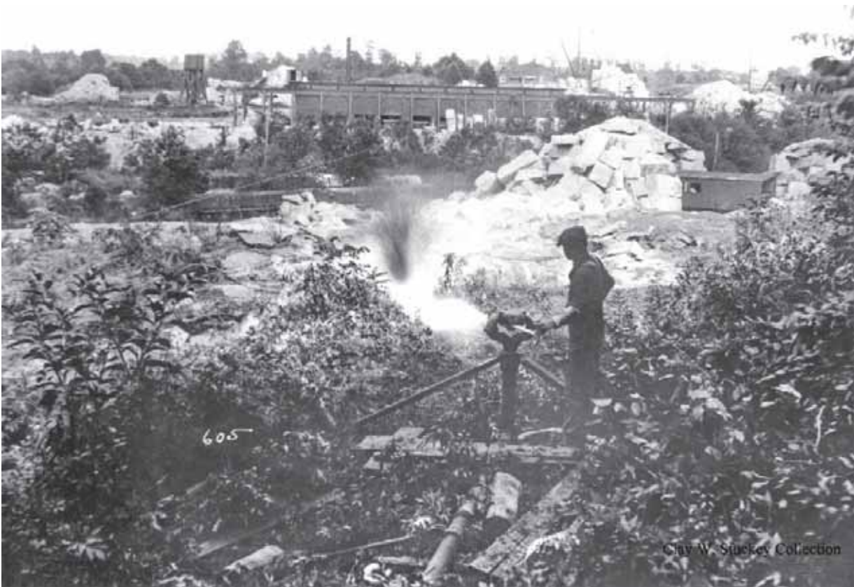
Fig. 15 The Vernia Mill (old Consolidated No. 1) is in the background and in the foreground a workman is removing earth overburden with high powered water.
