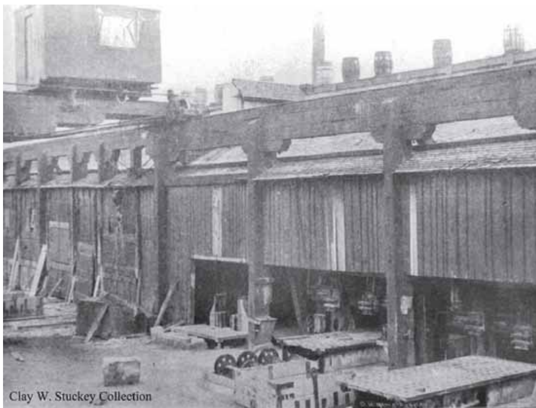
Fig. 268 From an 1895 issue of Stone magazine comes this picture of "THE HALLOWELL STONE CO.'S MILL, SHOWING PLANERS AND HEADERS." Note barrels of water for extinguishing fires.
