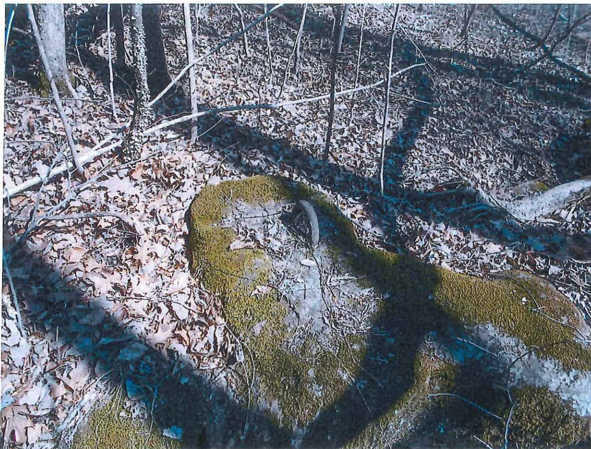
Fig. 1 Anybody walking through the dense woods looking for a quarry and running across something like this can rest assured that the quarry is close by. This is an anchor for a guy wire that would have supported a derrick.
