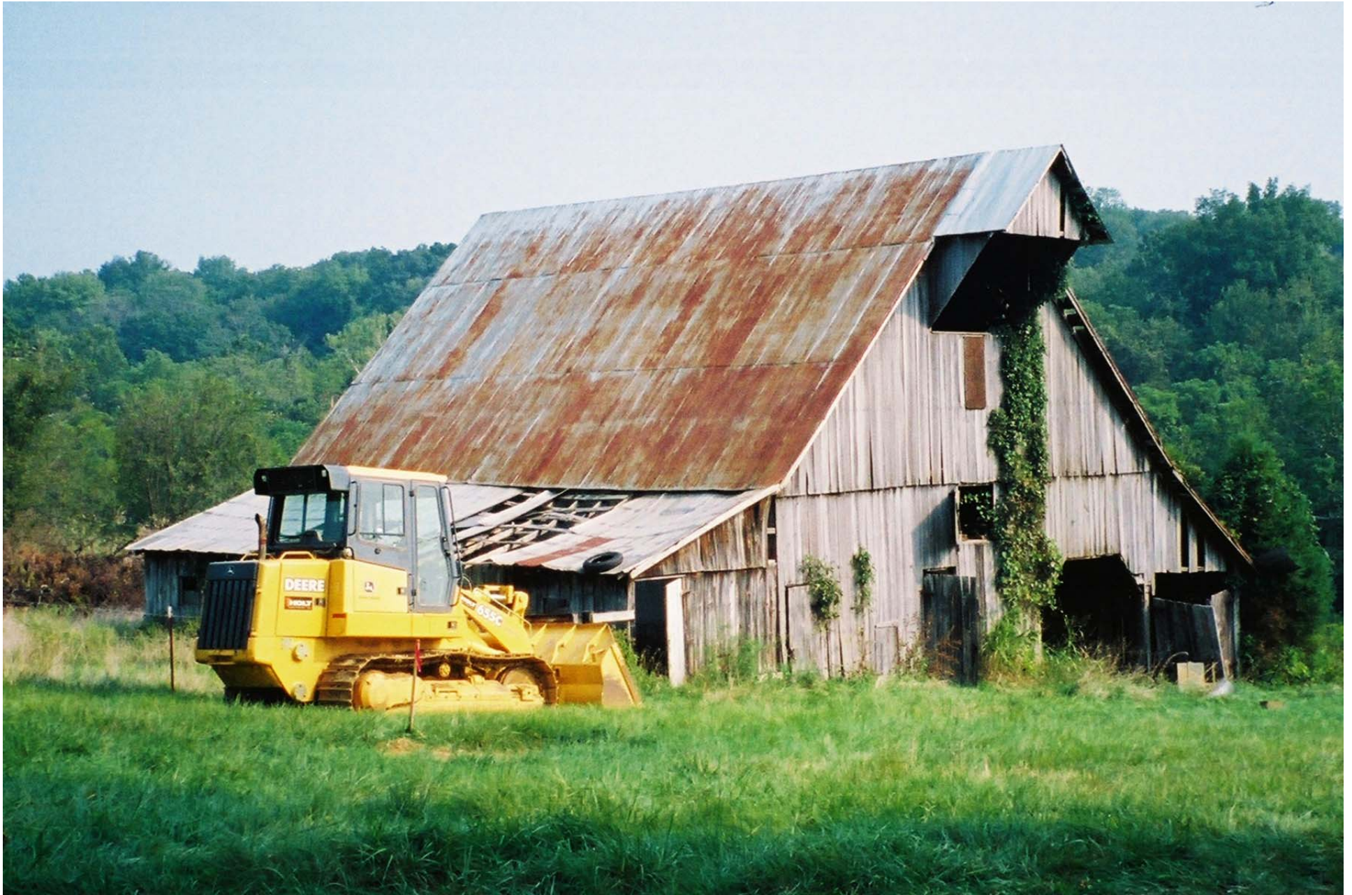
The Ketcham barn was threatened with demolition. The County carefully dismantled and moved the timber posts and beams to save this pre-Civil War structure. It was built of hewn timbers of poplar and other trees cut from virgin forest. The timber framing is stored while the County plans for the barn's "raising" -- reconstruction. The barn will be rebuilt in a county park, to be used for day camps, family reunions, picnics, and shelter, as well as for interpretive historic displays. (Photo by Cheryl Ann Munson)
