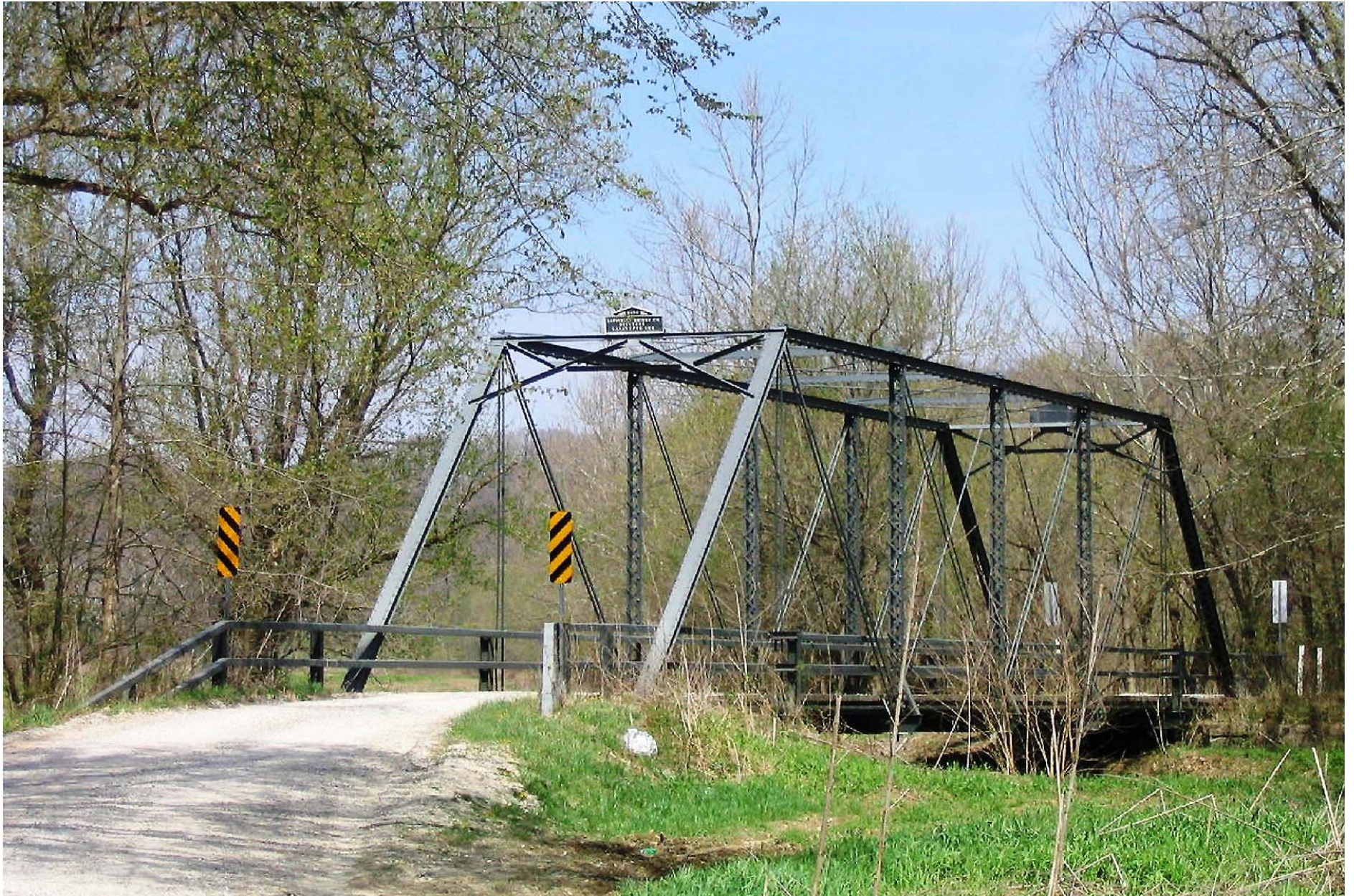
Friendship Road Bridge is an example of a Pratt-through Truss style. It was built in 1898 northwest of Bloomington, abandoned in 1947 when a new road was built, relocated to Friendship Road in 1948, and restored by the County in 2003. The County received a historic preservation award in 2004 from the Bloomington Historic Preservation Commission, for the restoration they accomplished. The County Historic Preservation Board, under its preservation ordinance, designated this structure for a historic zoning overlay to continue preservation for years to come. (Photo by Mary Pietsch Alexander)
