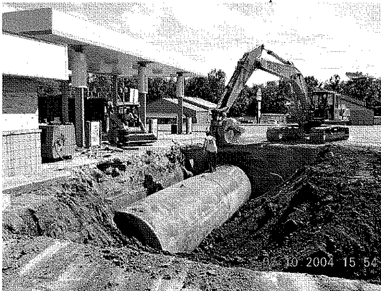
UNDERGROUND STORAGE TANK REMOVAL
