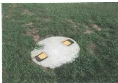
Two types of septic tank lids found on most septic systems installed after 1990
