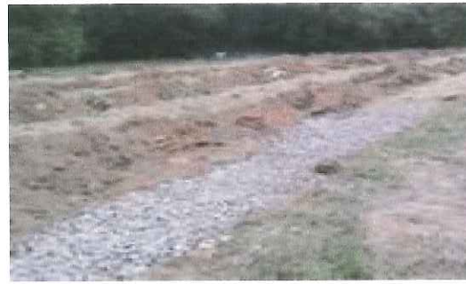
Trenches consisting of crushed stone and pipe
