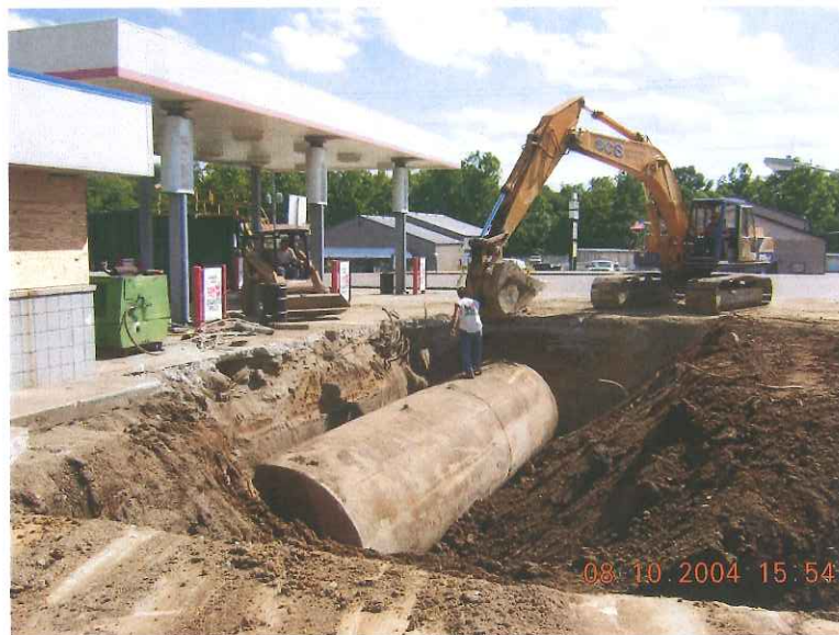
UNDERGROUND STORAGE TANK REMOVAL
