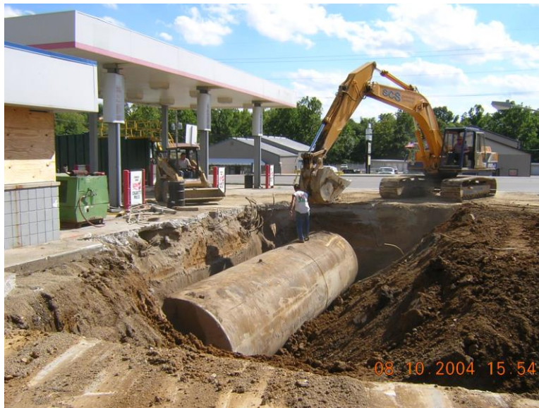
UNDERGROUND STORAGE TANK REMOVAL
