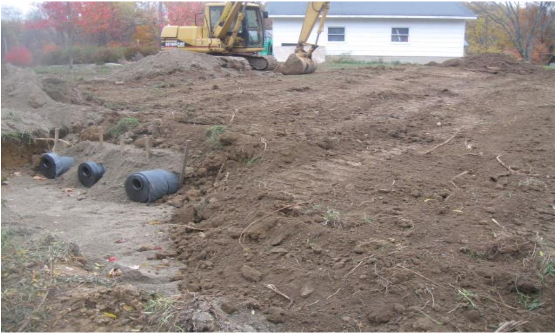
GEO-FLOW PIPE LEACHING SYSTEM
