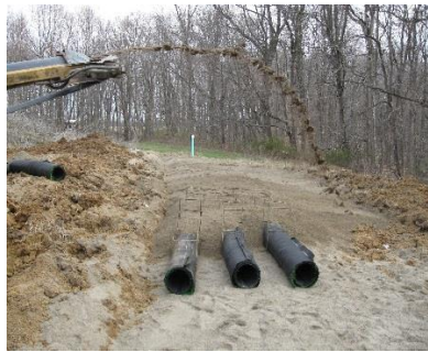
Placement of 6" sand and pipe
