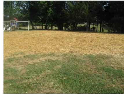
Final cover of 6" sand, 1 foot soil, with seed and straw
