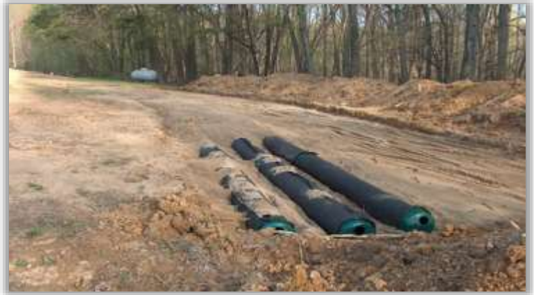
Installation of a normal three bedroom Presby Septic System
