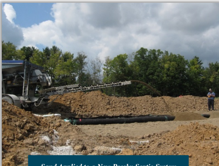
Sand Applied to a New Presby Septic System
