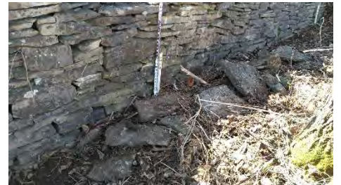
STA 0+20, close up collapsed stone.
