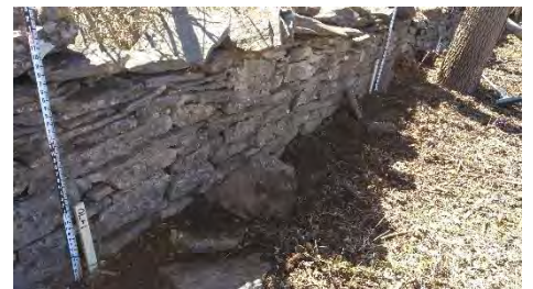
STA 1+70 to 1+80, collapsed stone.
