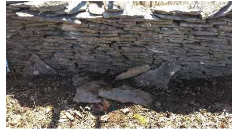
STA 1+20 to 1+30, collapsed stone.
