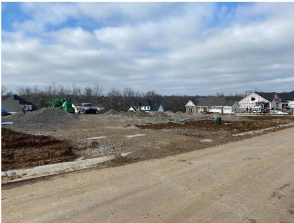
Significant accumulation of sediment beginning to build along road edges.
