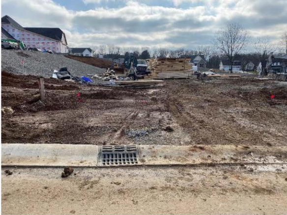
Inlet protections missing on Irie Ct.
