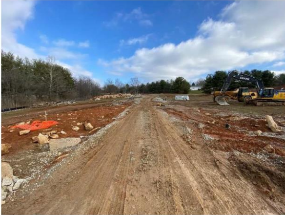
View from end of Phase 2, looking into Phase 3 & 4. Inadequate stone on access road.
