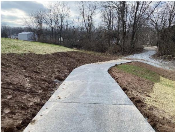
Trail access path from Irie Ct. Stabilize adjacent slopes as soon as possible to limit erosion and sediment transport onto path.
