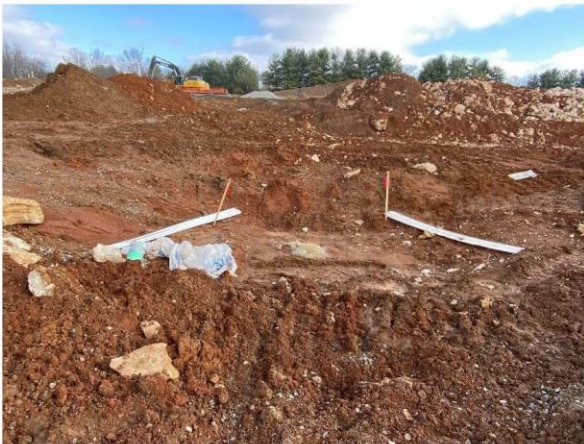
Protections on yard inlet between Lots 23 & 24 needs maintenance.
