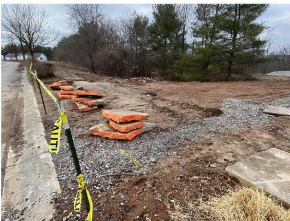
Phase 4 access off S College Dr. is adequately blocked and is not being used as a construction entrance. When work begins in Phase 4, adequate stone should be placed to prevent tracking from this road. Stabilization of areas disturbed for water line installation is inadequate. No perimeter controls are in place for Phase 4.
