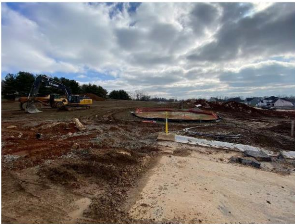
Sinkhole remains adequately protected. Repair silt fence as needed. Street inlets at the end of Phase 2 are adequately protected.
