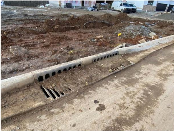
Inlet protections missing or severely damaged. Remove accumulated sediment and replace inlet protections.
