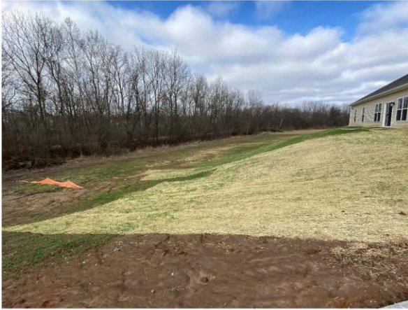
View toward rear yard of Lots 61 & 60. Slopes adequately stabilized. Additional seed and stabilization will be necessary in spring on low point.
