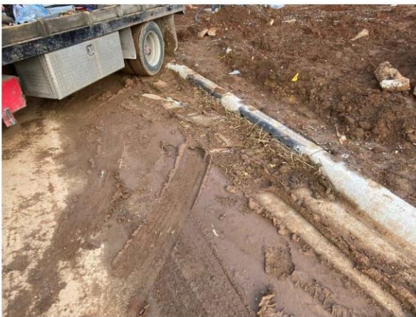
Accumulated sediment has overwhelmed the inlet protections.
