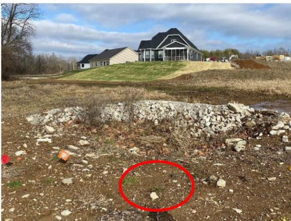
Yard inlet protection needs maintenance.
