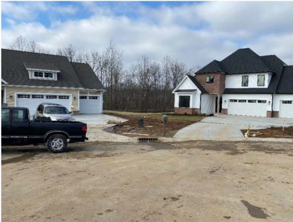
Inlet protections missing on Irie Ct.
