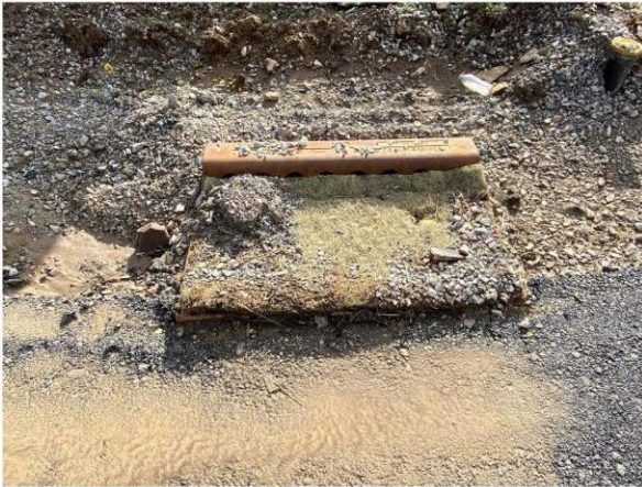
Inlet protections on That Rd at Rogers need maintenance.
