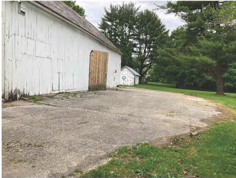
The side exterior of the barn. Note the siding that is beginning to deteriorate
