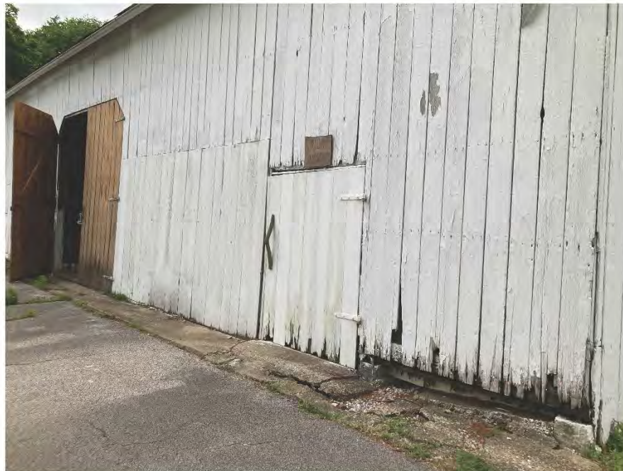
The side exterior of the barn. Note the siding that is beginning to deteriorate
