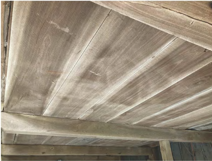
Interior barn details like the wide poplar boards and the wooden pegs in the beams
