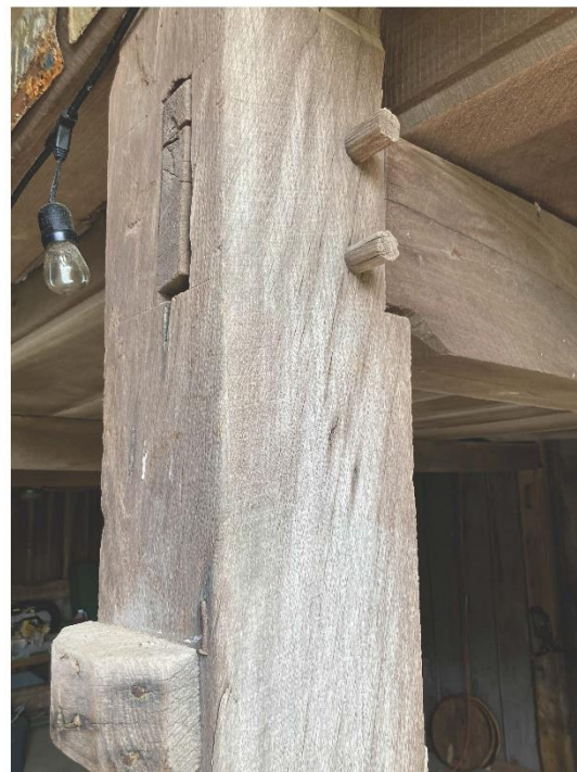
Interior barn details like the wide poplar boards and the wooden pegs in the beams
