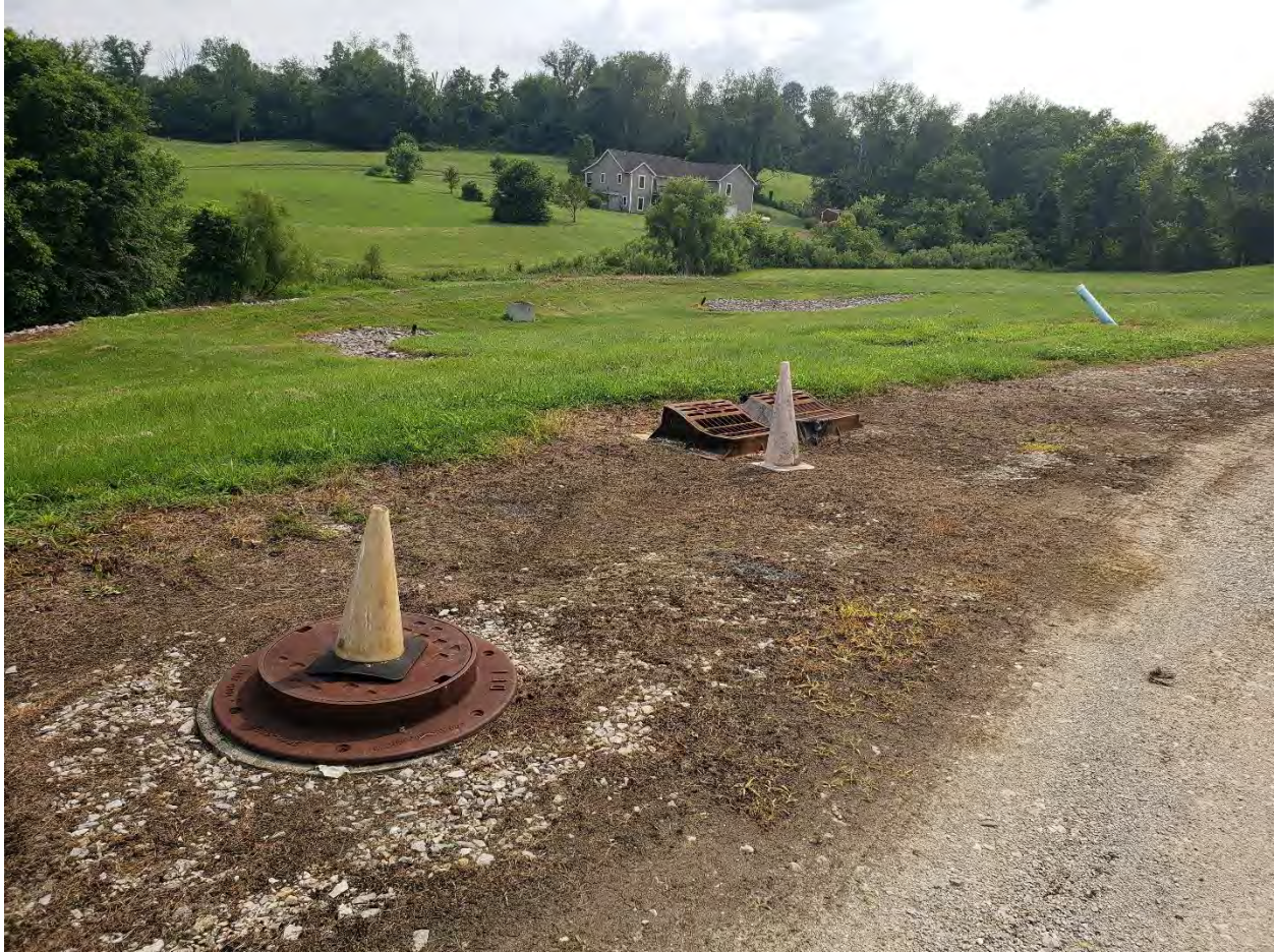
Manholes, storm sewer, sanitary sewer, and retention ponds are installed.
